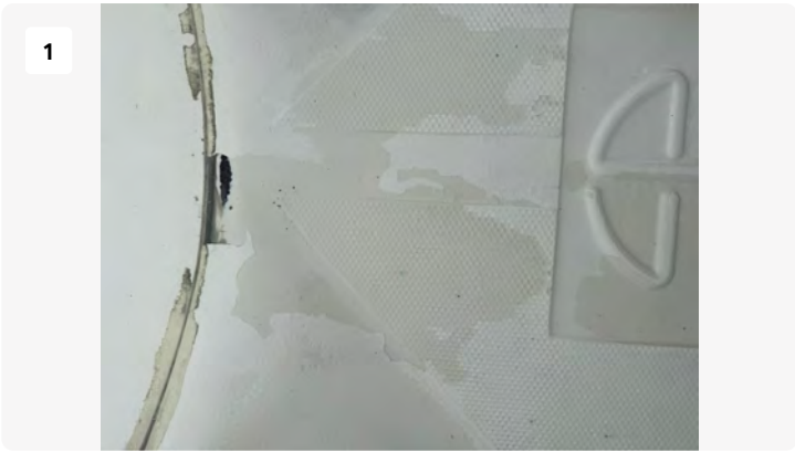
Failed and thinning gelcoat.
