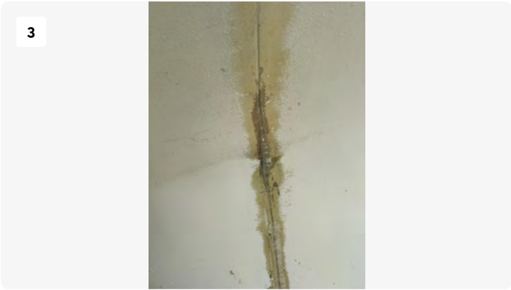
Up-close of previous coating and surface caulk.
