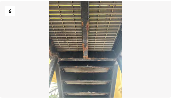
Underside of slide tower:
