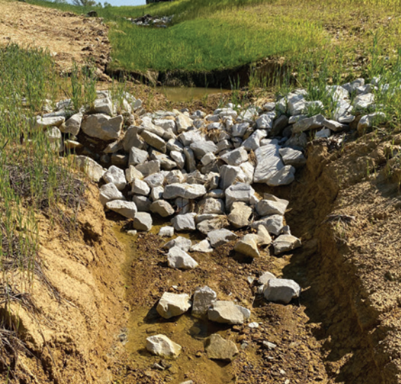
ShearForce10 installation in channel vs rock riprap.
