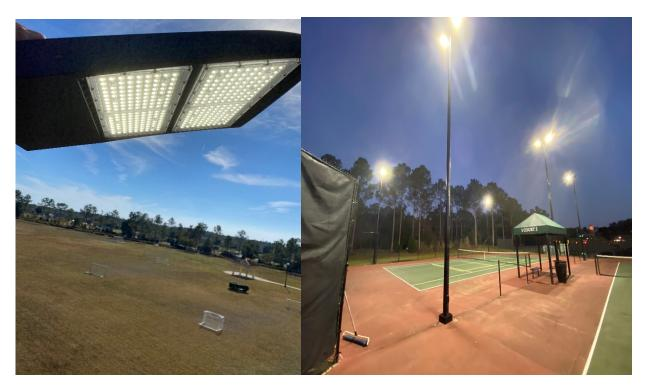
Replaced 12 old ballast sodium light fixtures on tennis courts with new LED light fixtures
