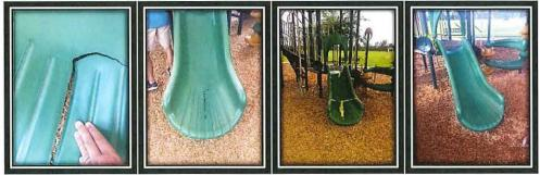
The 3ft kiddie slide at the amenity playground cracked and ripped open causing a dangerous sharp edge. The new slide was ordered and installed.
