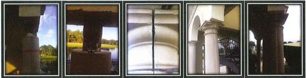
All the columns on ground level at the slide tower were opened and secured with metal brackets. All were glued and caulked back together.
