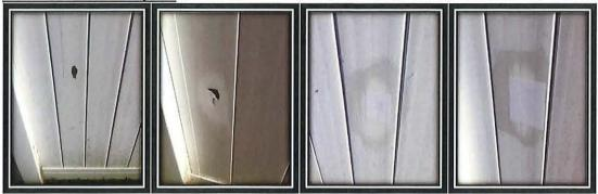
A resident called saying the landscapers damaged their fence. I asked Duval and they could not recall causing the damage. I ordered a patch kit for pvc fence and repaired the holes.
