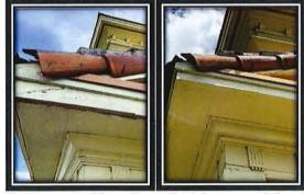
Cutting out old caulk on the trim around the slide tower, re-caulk and paint all the way around.
