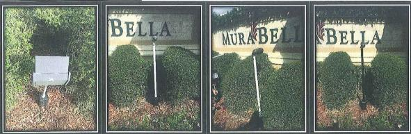
The old spot lights were rusting out and allowed moister to get in. The bulbs kept blowing out, we replaced them with a led fixture from Home Depot.
